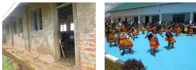
St Thereza Bwendero Primary School before (left) and after (right) redevelopment.
