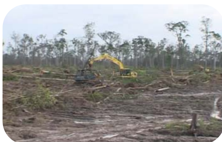
Land clearing by mechanical means
