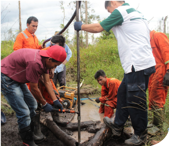
Tubewell construction as part of fire suppression efforts in Central Kalimantan.
