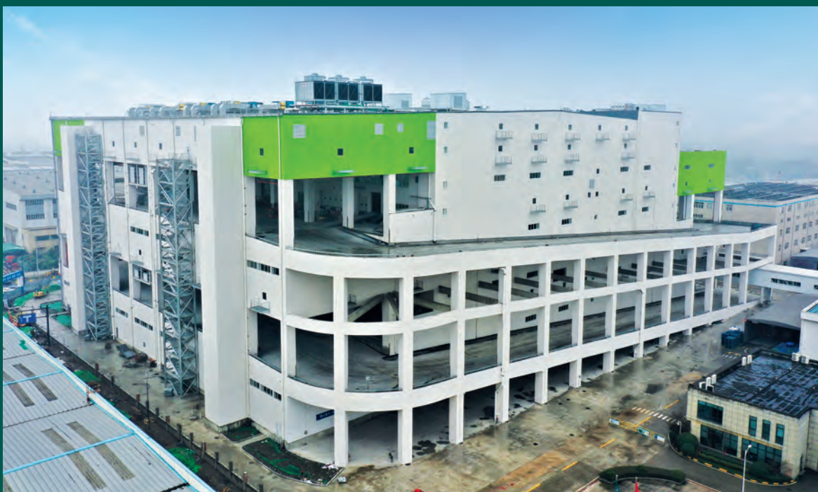
Central kitchen in Hangzhou, China.
