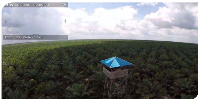
Aerial view of fire tower
