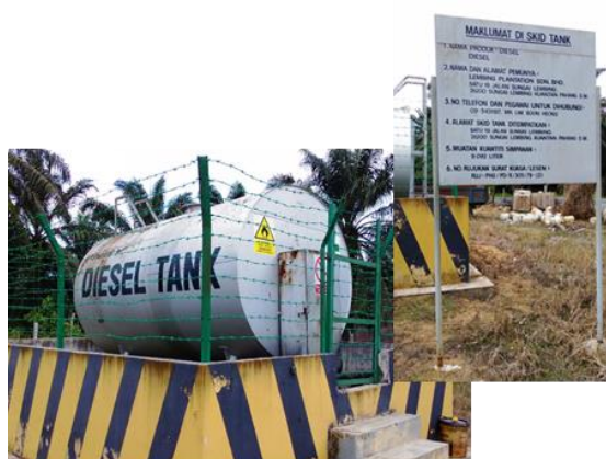
Figure 3 Containment bund for hazardous storage with proper label.
