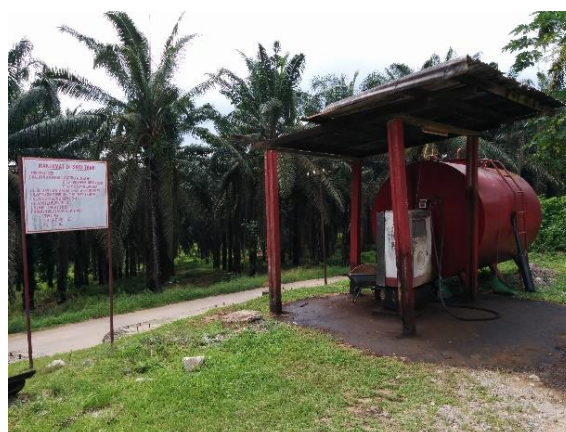
Figure 4 Diesel skid tank placed with no containment bund.
