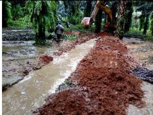
Figure 4: Work to divert the course flow of the POME
