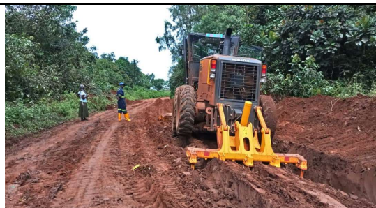
Figure 6: Regrading efforts to fix the connecting roads
