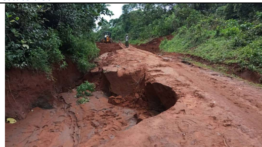
Figure 5: Damaged parts of the connecting road to the community due to overflow
