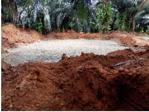
Figure 1: An emergency pond constructed to receive POME overflow
