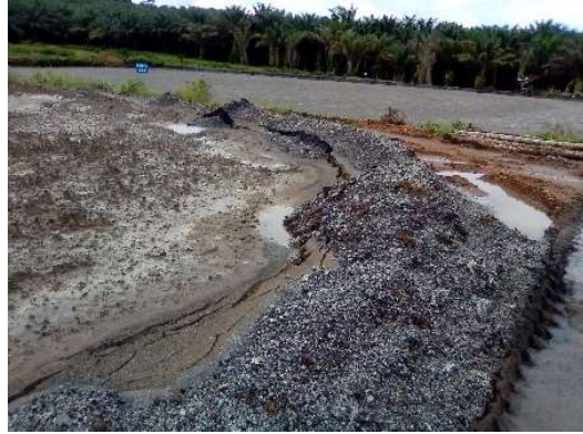
Figure 2: Overflow of the POME treatment ponds
