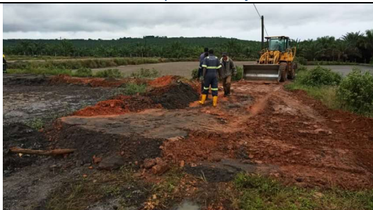
Figure 7: Blocking of the effluent using wheel loader
