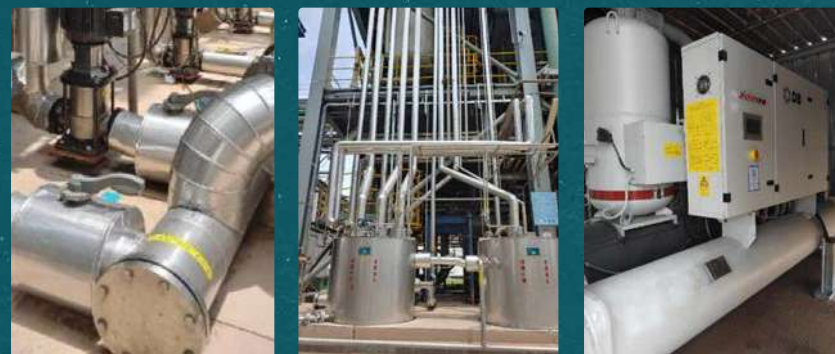
All Wilmar oleochemical plants in China have been upgraded to the Chiller Vacuum System, comprising of the Condenser System (top), Circulation Pump System (bottom left), Hot Well Unit (bottom center) and the Chiller Unit (bottom right).
